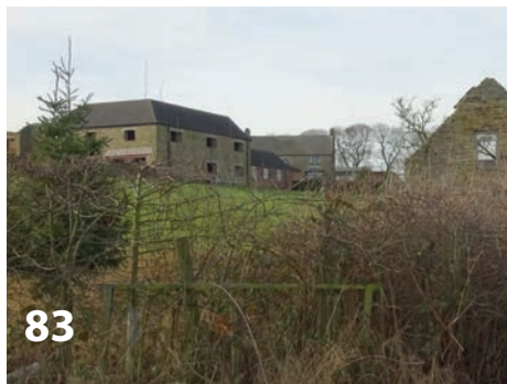
Biggin Farm, Chesterfield Road
