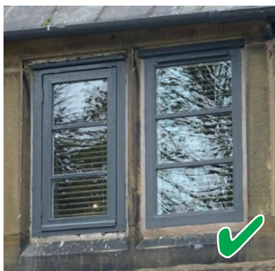
Painted timber flush casement
