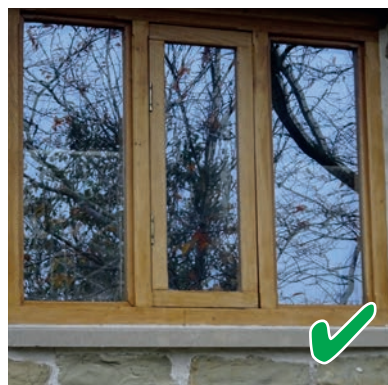
Varnished hardwood flush casement
