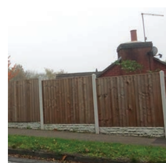
Very high panel fencing especially with concrete posts and bases.
