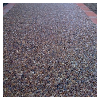
Permeable resin bound gravel.
