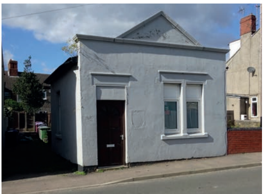
A former bank converted to a dwelling.
