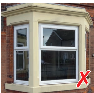
UPVC storm casement windows with 45 degree welded corner joints in brilliant white.
