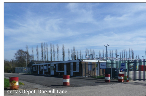
Site of Britain's First Inland Oil Well
