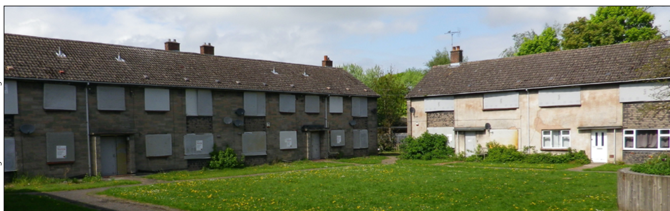
Flats off High Street: soon to go
