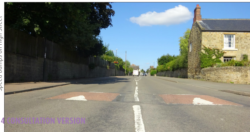
Speed bumps on High Street
