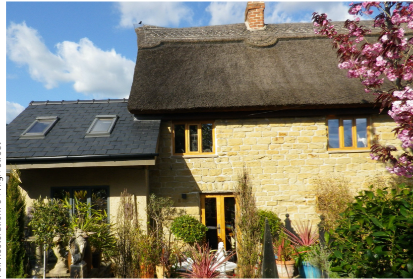
Full Restoration: 64 High Street
