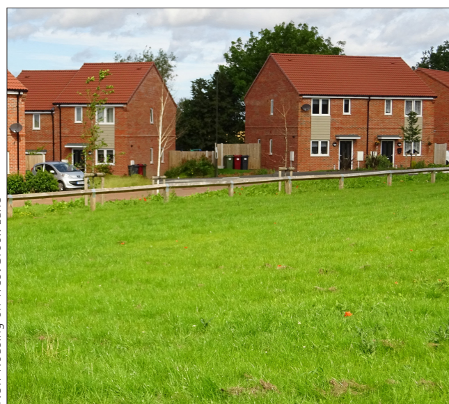
New Housing on West Brook Lane
