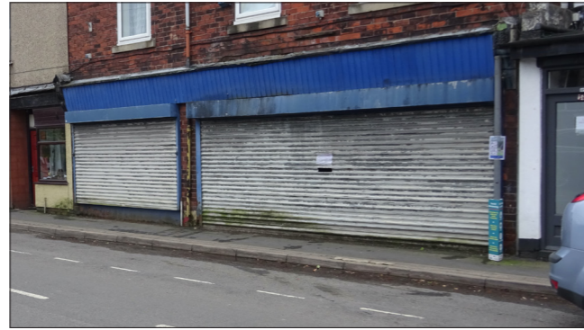
Unattractive shop front shutters
