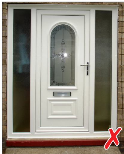
Brilliant white UPVC with a thick frame and 45 degree welded corner joints
