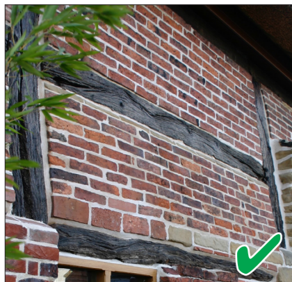
A few buildings in Tibshelf are of a medieval construction: oak timber frames with infills of brick.
