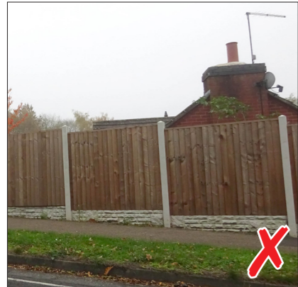
Very high panel fencing especially with concrete posts and bases
