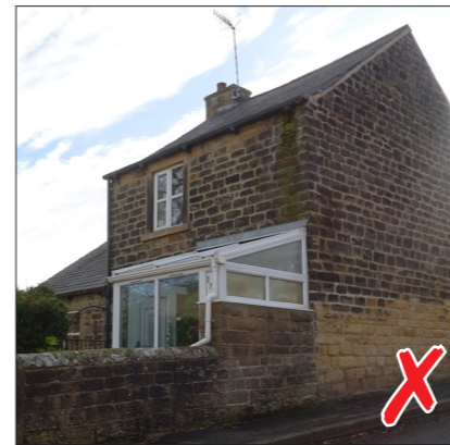
Above: Bad design and use of inappropriate materials and colours.
