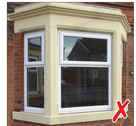
UPVC storm casement windows with 45 degree welded corner joints in brilliant white
