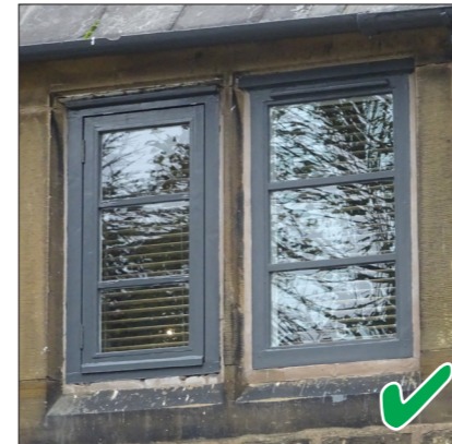
Painted timber flush casement
