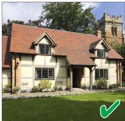
New build timber framed house with rendered infill panels.
