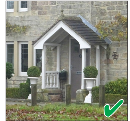
An attractive open porch which compliments the house.
