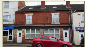
Private Housing converted from shops C3a
