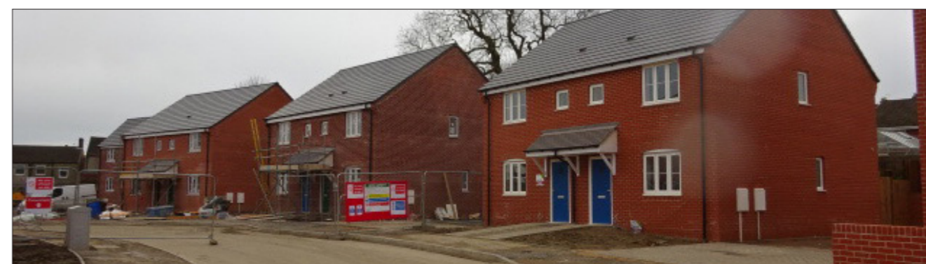
New Build on Mill Farm Drive
