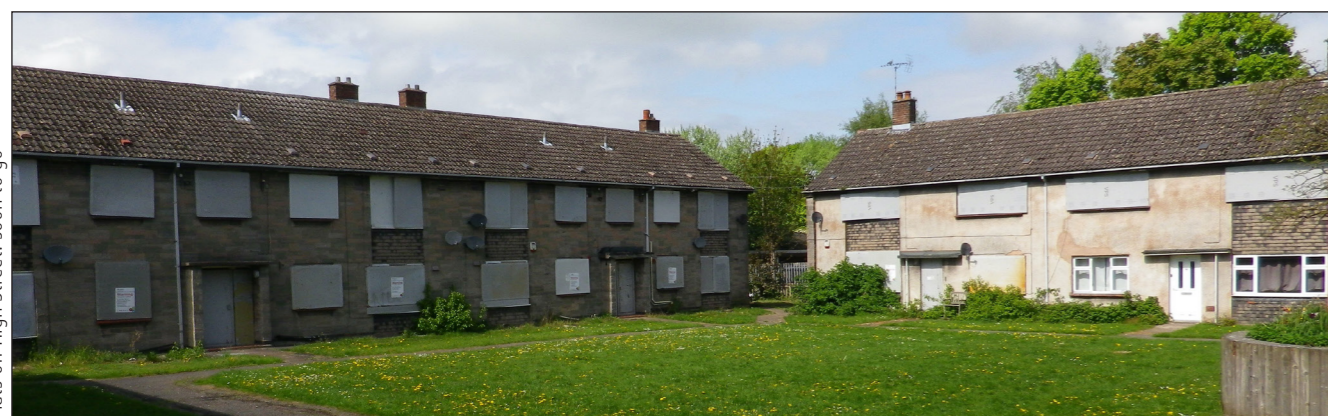
Flats off High Street: soon to go
