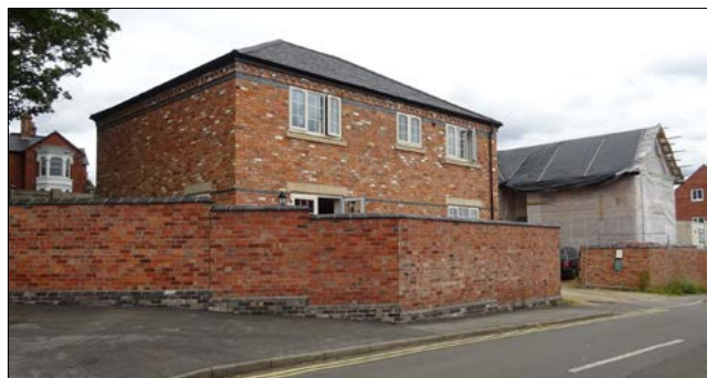
New Housing on Hardwick Street
