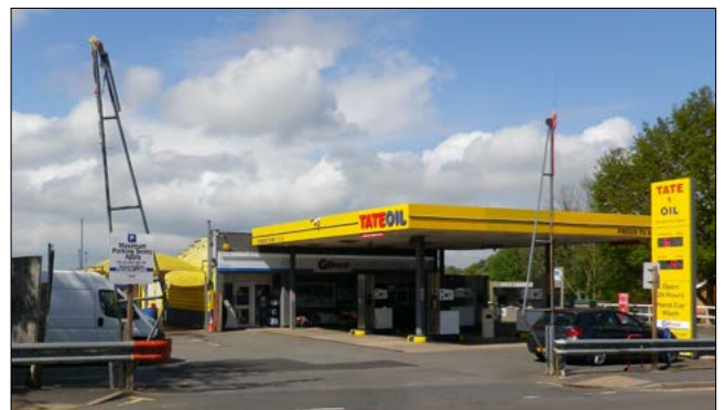
Filling Station, High Street
