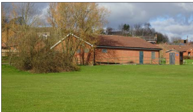
Sports Pavilion, Shetland Road
